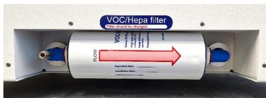
Figure 12.3 Filtre VOC/HEPA correctement installé
